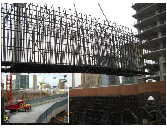
Pre-assembled beam being lowered into position after just-in-time delivery
