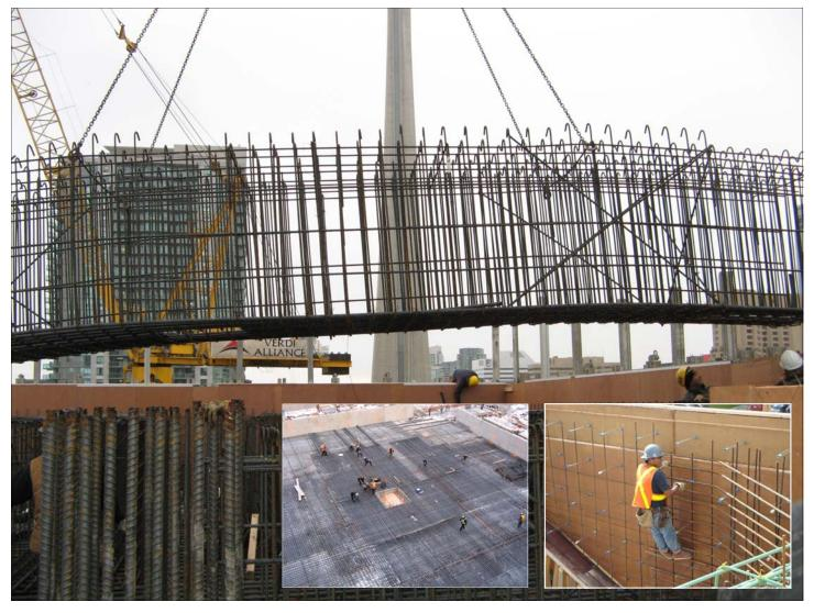
the project had fallen behind. The only way to speed up construction was to pre-assemble the columns and beams offsite and deliver on the same day they were ordered. There was no room on site to allow for pre-assembly of beams or columns. Onsite rebar tying was undertaken by SRI Installations.
