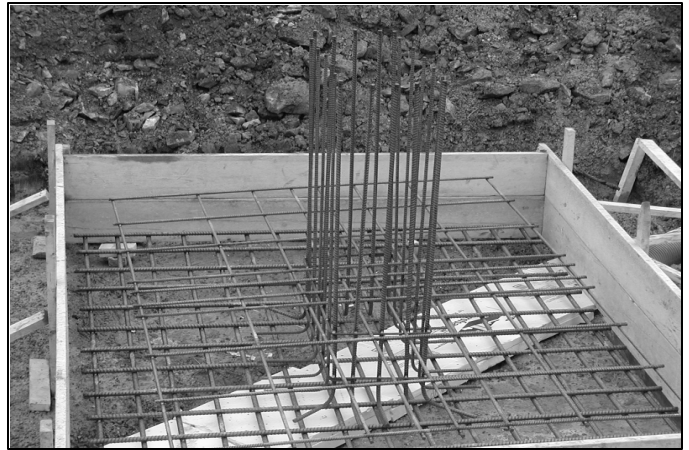
Pre-welded footing and pier reinforcement.
