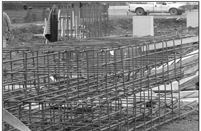
Pre-welded assemblies for electrical duct banks
