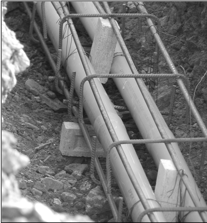
Pre-welded cross bars to ensure the plastic conduit would be spaced away from the bottom of the rebar cage.
