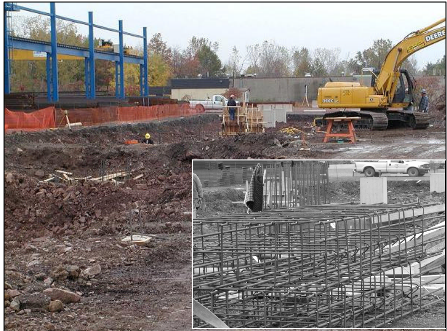
Site preparation for placement of pre-welded footings, piers and conduit ducts.
