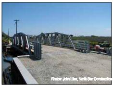
Specially designed superstructure placed on precast abutments with pre-welded stainless steel reinforcement.
