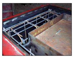
Pre-welded cage placed in transformer formwork.
