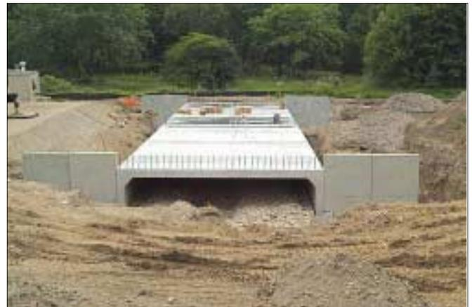
Installed precast bridge and wing wall units. Exposed rebar dowels were supplied pre-welded as part of the reinforcing cage assembly
