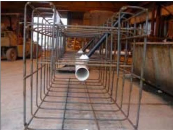
Pre-assembled footing reinforcing cage; complete with cross supports for the post-tensioning ductwork
