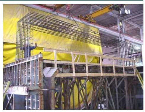
Bridge reinforcing cage being lowered into the casting mould
