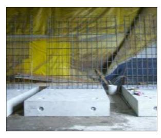
Precast Wing Wall: L shaped units ready for secondary pour of wall sections
