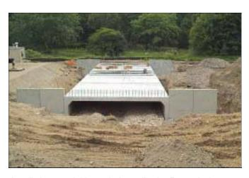
Installed precast bridge and wing wall units. Exposed rebar dowels were supplied pre-welded as part of the reinforcing cage assembly
