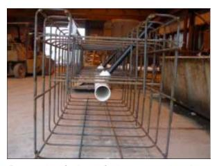
Pre-assembled footing reinforcing cage; complete with cross supports for the post-tensioning ductwork
