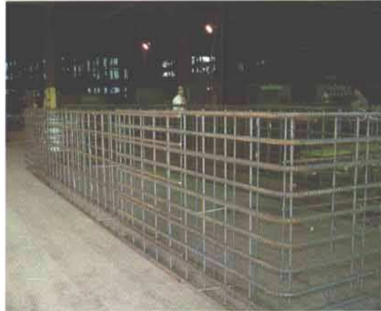
Pre-welded reinforcing assembly for Quick Span mould.
