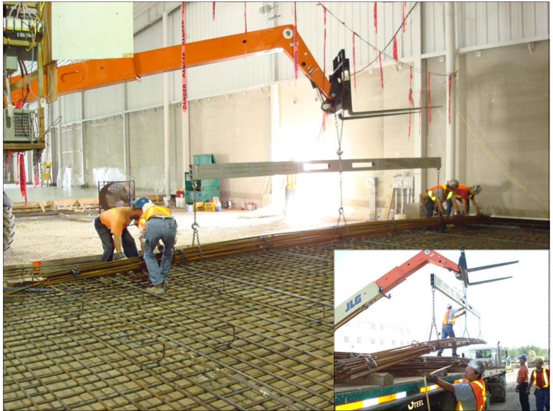
Pre-assembled carpet roll removed from flatbed and positioned inside Building 3
