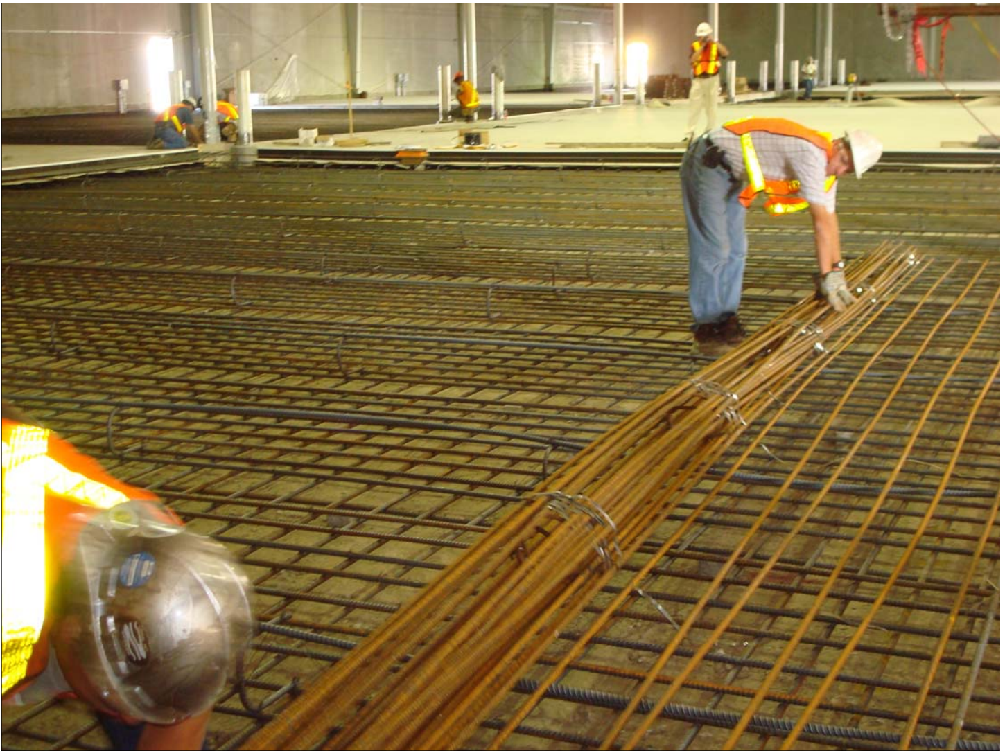
Pre-assembled mat rolled into position to accommodate poured-in-place floor construction for supporting dry storage containers
