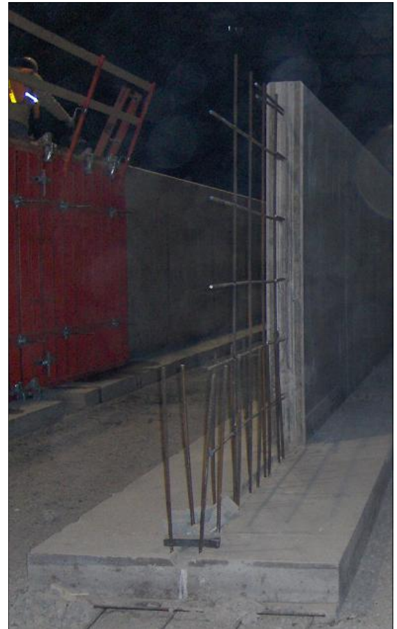
Section of poured-in-place compost channel
