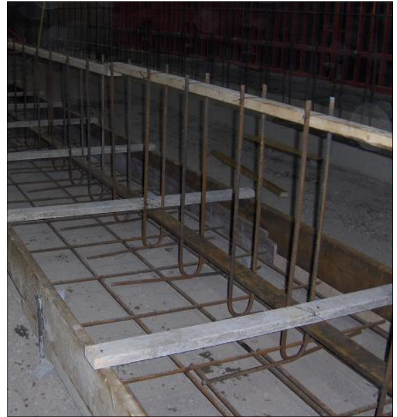
Positioned assemblies to accommodate rebar mats
