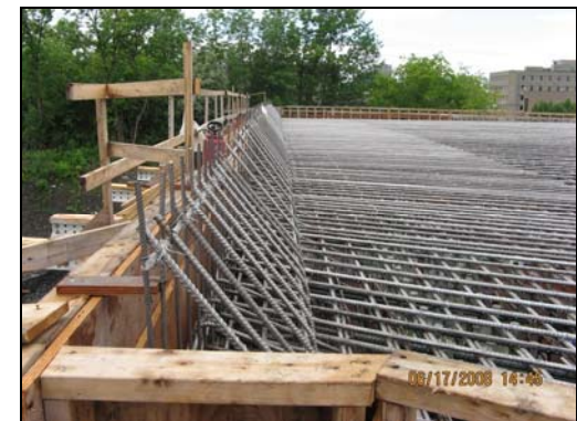
Concrete decks and barrier walls reinforced with Alloy 2205 stainless steel.
