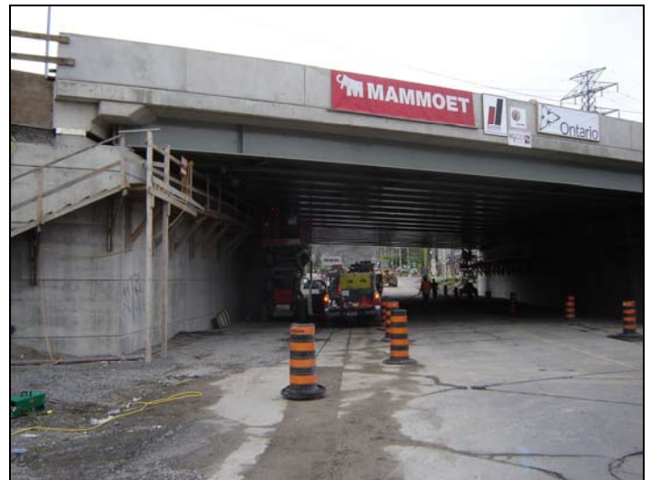
New precast structure set in place within 24 hours.
