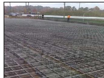
Stainless steel deck on Highway 409 Photo: Salit Steel
