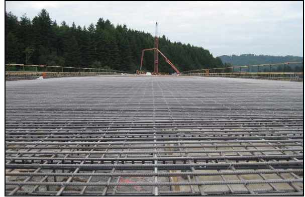
Deck comprised of Type 2205 duplex stainless steel. Photo: Dixon Steel
